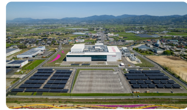
Solar panels at the Fukuoka Kurume factory (Japan)
