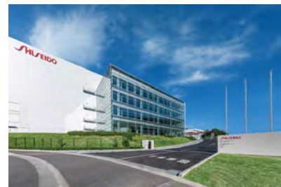
West Japan Distribution Center
