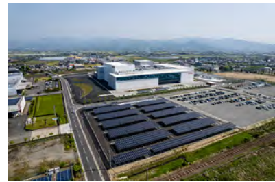
Solar panels at the Fukuoka Kurume factory (Japan)
