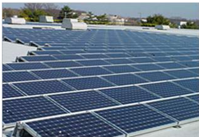
Phase 1 installation (fixed-tilt system)
