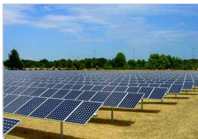
Phase 2 installation (solar tracking system)
