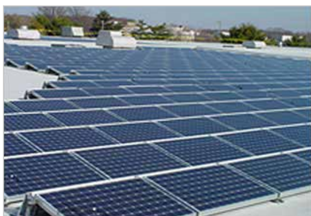
Phase 1 installation (fixed tilt system)
