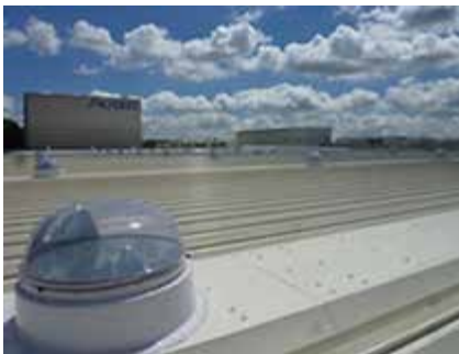
Solar-powered lighting (rooftop)
