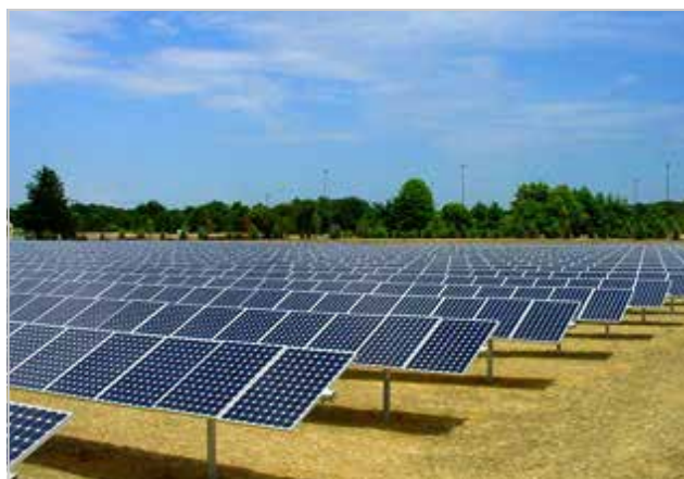
Phase 2 installation (solar tracking system)
