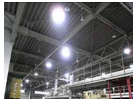
Solar-powered lighting (inside storage facility)
