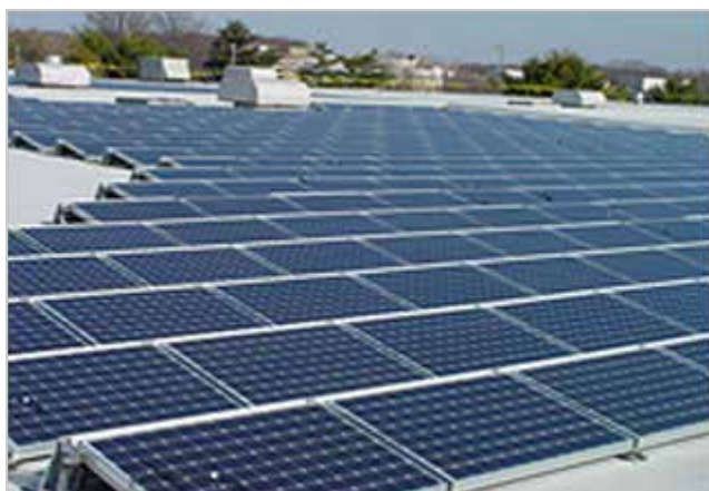
Phase 1 installation (fixed tilt system)
