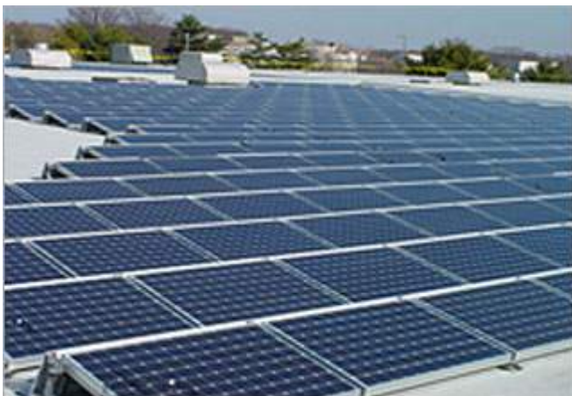
Phase 1 installation (fixed tilt system)
