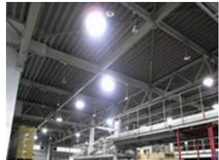
Solar-powered lighting (inside storage facility)
