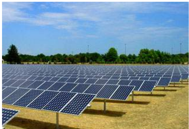
Phase 2 installation (solar tracking system)
