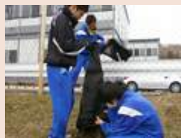
Installing snow guard net on poles
