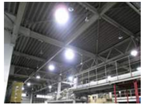
Solar-powered lighting (inside storage facility)
