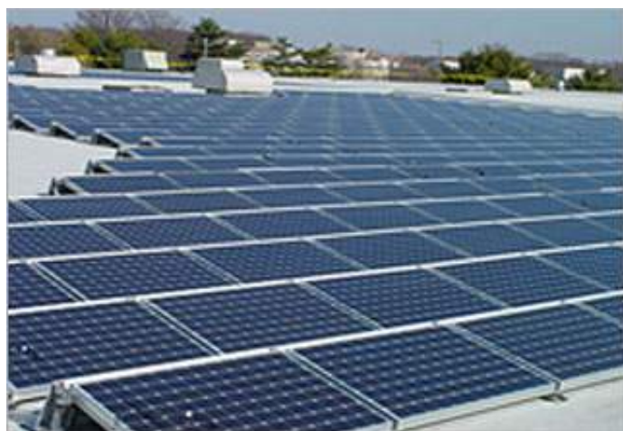
Phase 1 installation (fixed tilt system)
