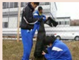
Installing snow guard net on poles
