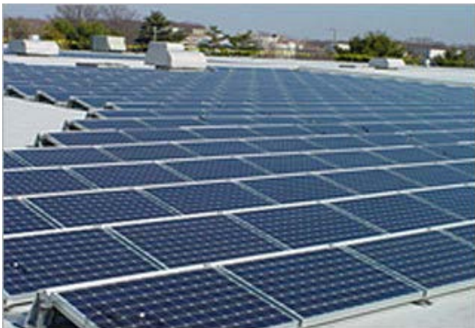
Phase 1 installation (fixed tilt system)
