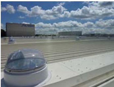
Solar-powered lighting (rooftop)
