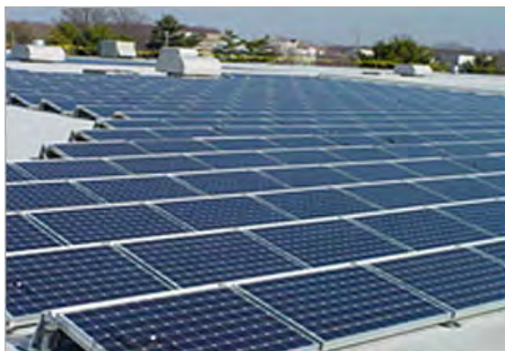
Phase 1 installation (fixed tilt system)
