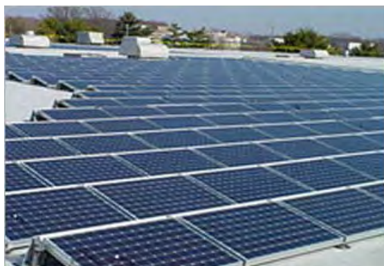
Phase 1 installation (fixed tilt system)
